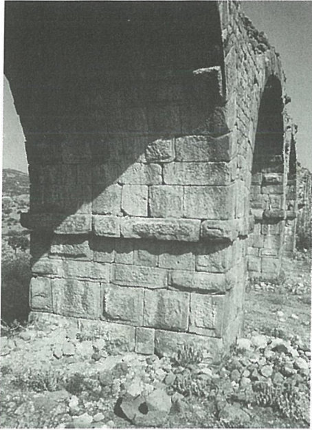
Figure 3. A stone (trachyte) anchor block of the lead pipe inverted siphon of Pergamon, from the 2nd century BC, resisting a maximal pressure of 190 m and supplying the acropolis; and the later aqueduct, from the 1st century BC/AD, supplying less elevated parts.
