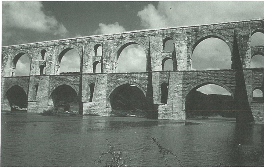
Figure 7. The 35 m high Mağlova aqueduct on the Kırkçeşme water conveyance system to Istanbul, constructed by the Architect Sinan in 1564.
