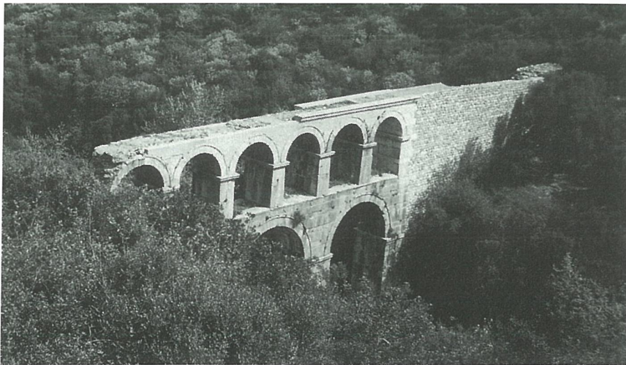
Figure 4. The 16 m high Sextilius-Pollio aqueduct on the Marnas water conveyance system to Ephesos, from 4–14 AD.
